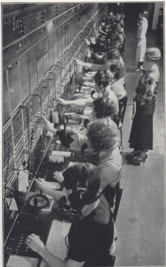
These Long Distance operators have scores of cities at their finger-tips and timing devices at each right hand which stamp the length of your conversation on the record of your call.
