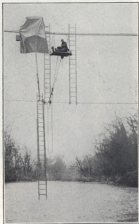
Splicing telephone wires where the cable highway crosses a river.
