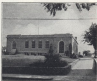
A repeater station where vacuum tube amplifiers are installed on long distance circuits to maintain volume and quality.
